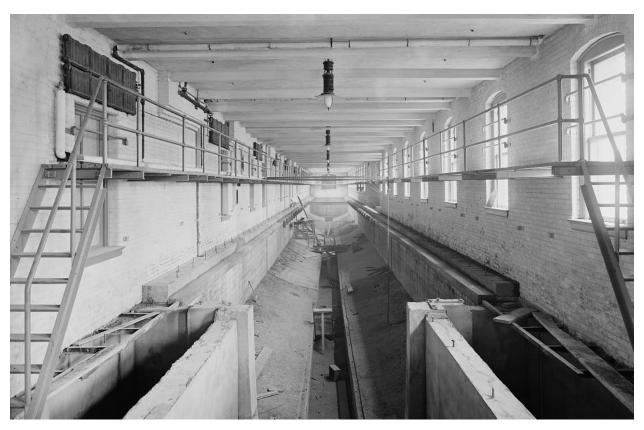
$\ldots$  and this naval tank, where students tested the hydrodynamics of model ships.
