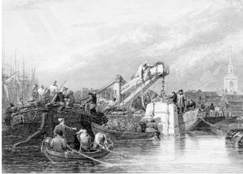
The diving bell in which Humboldt descended with Brunel to the bottom of the Thames to see the construction of the tunnel
