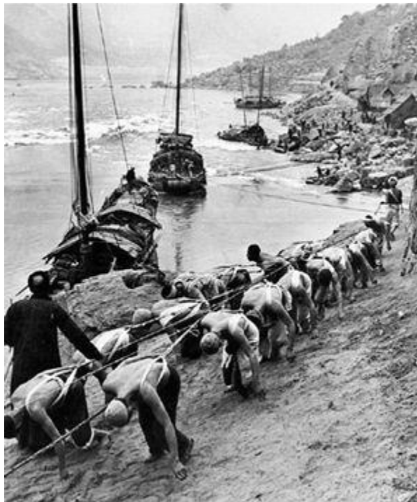
Gangs of trackers bending to their work towing a riverboat along the banks of the Yangzi River. Sixteen trackers are seen in the gang in the foreground, which is pulling the second vessel from the left. The photograph was taken in the 1930s, but little had changed in the millennium since Zhang Zeduan painted Along the River During the Qingming Festival eight centuries before (see insert, figure 11 ). Photograph by Dmitri Kessel; courtesy of Life magazine.
