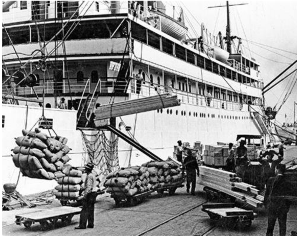
Stevedores, or longshoremen, off-loading cargo from a ship on the Mississippi River at New Orleans in the 1940s. While deck cranes provided some degree of automation, handling cargo remained a labor-intensive occupation, and a total of thirteen people can be seen in this tight picture of a relatively small ship. Within twenty years, the nature of commercial shipping had changed beyond all recognition, as is easily seen in the aerial photograph of the port of Singapore (see insert, figure 24 ). Courtesy of the Louisiana Digital Library.
