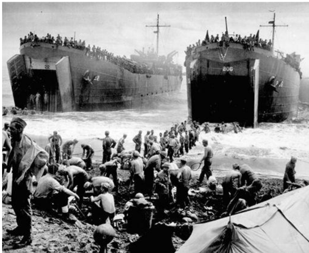
Two Coast Guard-manned Landing Ship, Tank (LSTs) with their bow doors open to the beach on Leyte Island, the Philippines, in 1944. Sailors are laying down a sandbag causeway from
